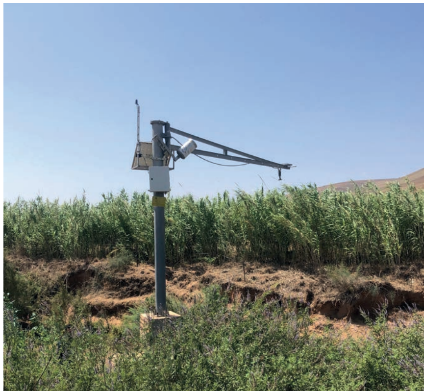
Station radar d'annonce de crue Ait Mouted.
